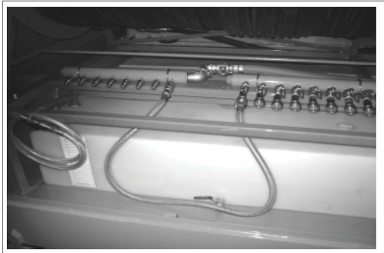
Fig. 43 SUPPLY MANIFOLD VALVES (SIMULATED)
