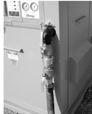
*Figure 6 - two inch circulation line to water heater cabinet connection*
