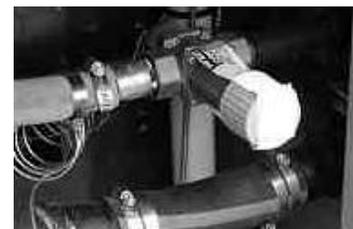
Figure 25 - thermostatic control valve
