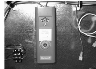
Figure 19 -U.S. high limit switch
