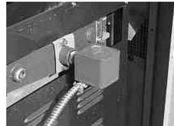
Figure 24 - water flow switch
