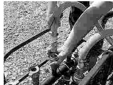
*Figure 8 - ¾", 1" and 1 ¼" circulation line to circulation manifold connection*
