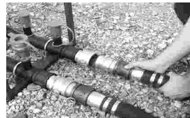
*Figure 7 - two inch circulation line to circulation manifold connection*
