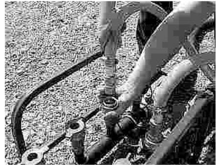
Figure 14 - connecting circulation lines to circulation manifolds
