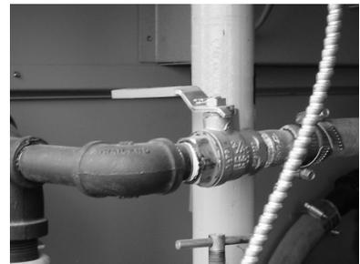
Figure 12 - air elimination valve
