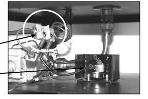
3. While the heater unit does not require a filter, the unit must be kept clean and the burner and pilot assembly must be kept free of dust and dirt to ensure optimal and safe operation at all times
