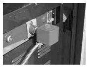
Figure 24 - water flow switch
