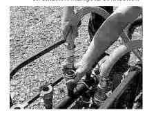
Figure  $8 - \frac{3}{4}$ ", 1" and  $1\frac{1}{4}$ " circulation line to circulation manifold connection
