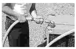
Figure 13 - connecting circulation lines to portable heat exchanger
