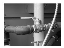
Figure 12 - air elimination valve
