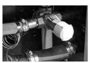
Figure 25 - thermostatic control valve
