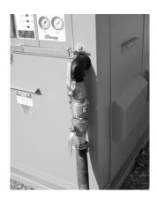
Figure 6 - two inch circulation line to water heater cabinet connection
