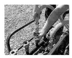
Figure 14 - connecting circulation lines to circulation manifolds
