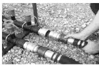
Figure 7 - two inch circulation line to circulation manifold connection
