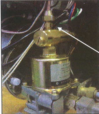
Picture 4 Inspection of the fuel pump
